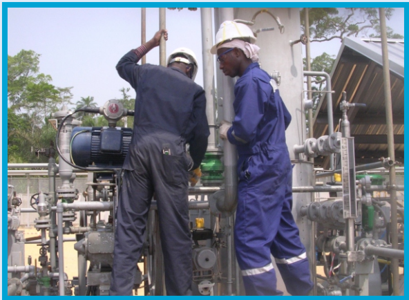
MECHANICAL SCREW MODIFICATION, WELDING WORKS (AGON WELDING) WITH CERTIFIED FITTERS/WELDERS AND EQUIPMENT, AT EPF PROJECT, GBARAN – UBIE.
