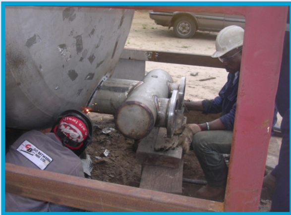
MODIFICATION OF STAINLESS NITROGEN TANK AND SKID.
