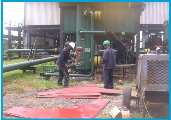
CUTTING OFF CORRODED PLATES AND REPLACEMENT OF NEW PLATES ON GAS COOLER HOUSING .
