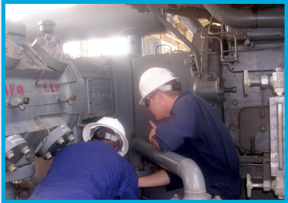
INSTALLATION OF VIBRATION SUPPORT, ADDAX GAS PLANT
