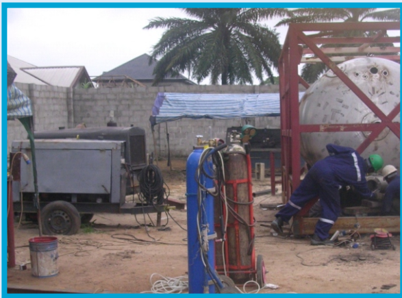
MODIFICATION OF STAINLESS NITROGEN TANK AND SKID.
