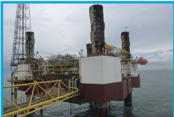
GAS COMPRESSOR HEAT X - CHANGER REPAIRS, ADDAX OFFSHORE
